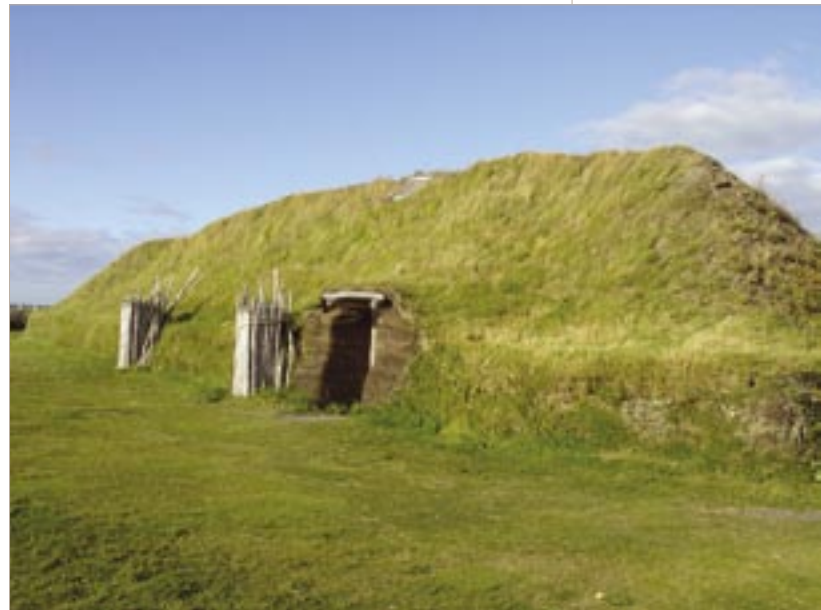
Throughout the North Atlantic, the Norse lived in houses made of sod, a readily available material which provided good insulation against cold winters.
